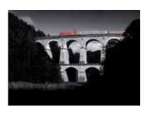
Example of an ancient, proven basic principle. Formation of compressive stress - avoidance of tensile stress
